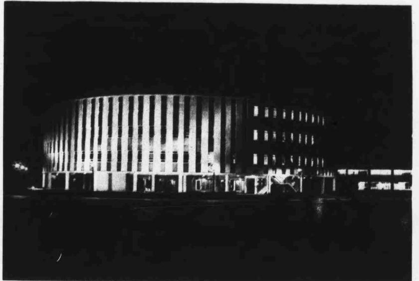
Harrelson Hall sits quietly at night with lights glowing all around. As State's only circular building, Harrelson is as unique as having no students wandering on the Brickyard.
