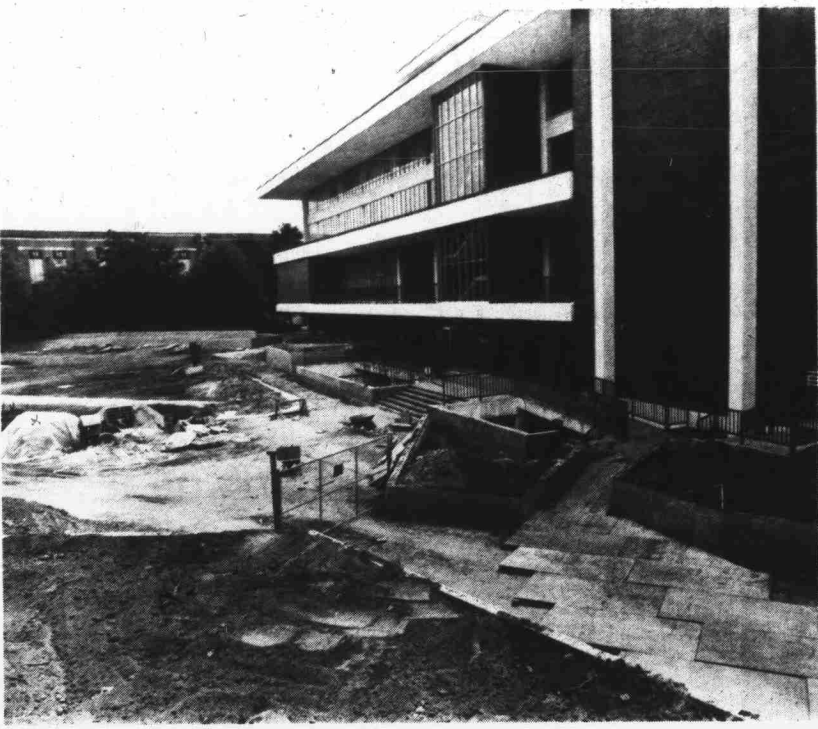
Landscaping of the University Student Center Plaza has progressed from a nice clean grassy area to a dirty, red clay filled area with newly rising walls
