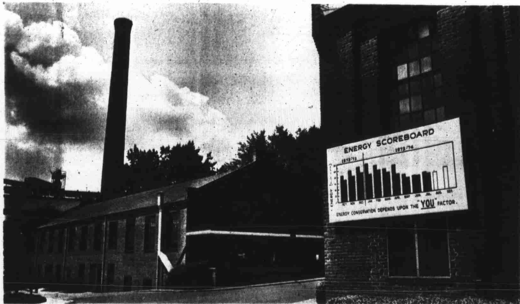
The energy scoreboard on the east wall of the park shops shows how well State is conserving energy. The dark lines indicate how much energy was used last year and the light lines show the energy used in the same month this year.
