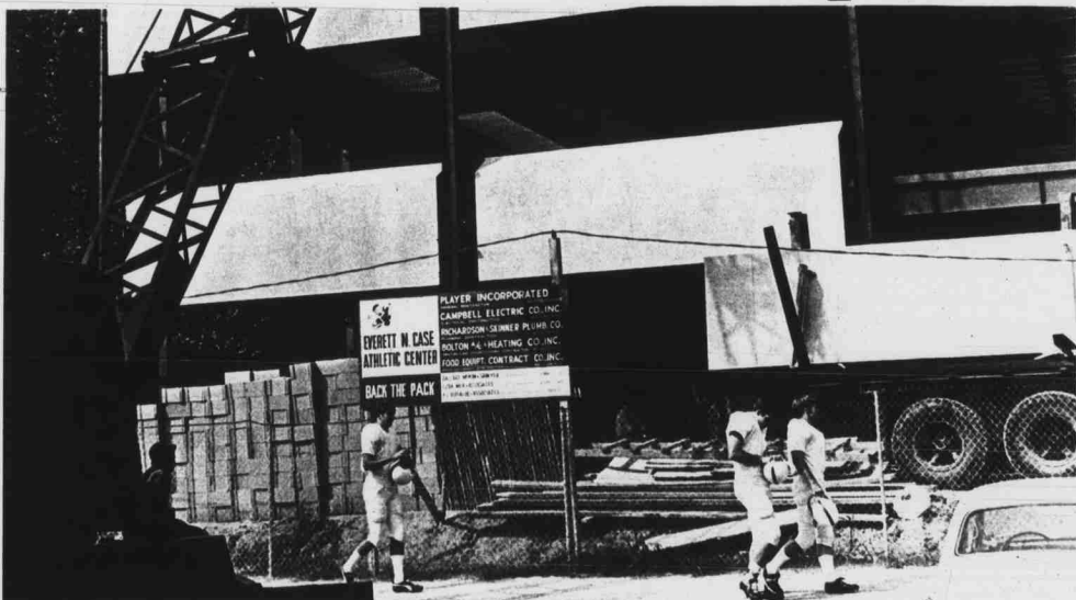
SOME OF STATE'S football players file past the front of the skeleton structure of the new athletic center. The new addition to State's rapidly growing complex is named in honor of the late Everette M. Case. —photo by Caram
