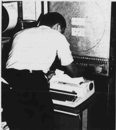
—photo by Wells "Hal 4096" lacks an interface for its keyboard. Meanwhile, its creator communicates by means of a panel of switches.
