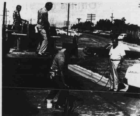
Physical Plant workers lay new cable to restore power to blacked-out Sullivan. The electrical service had faded at 9:10 Saturday night. —photo by Caram
