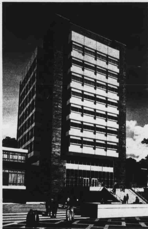
The new 11-story addition to the D. H. Hill Library will help increase its capacity to 1,100,000 volumes.
