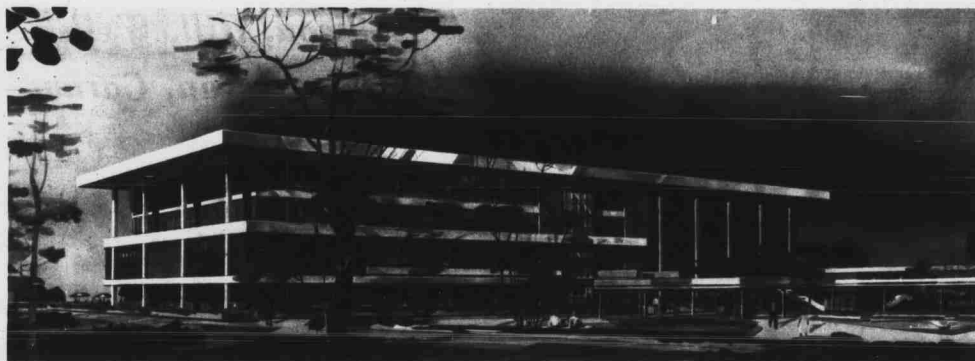
University center is the name given to the new Student Center now under construction. It is being paid for
