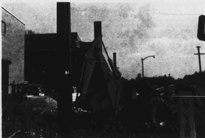
Staff Photo by Rob Westcott No, its not for another brick mall. It's the start of construction of a new $800,000 addition to Broughton Hall. Completion is set for next year.
