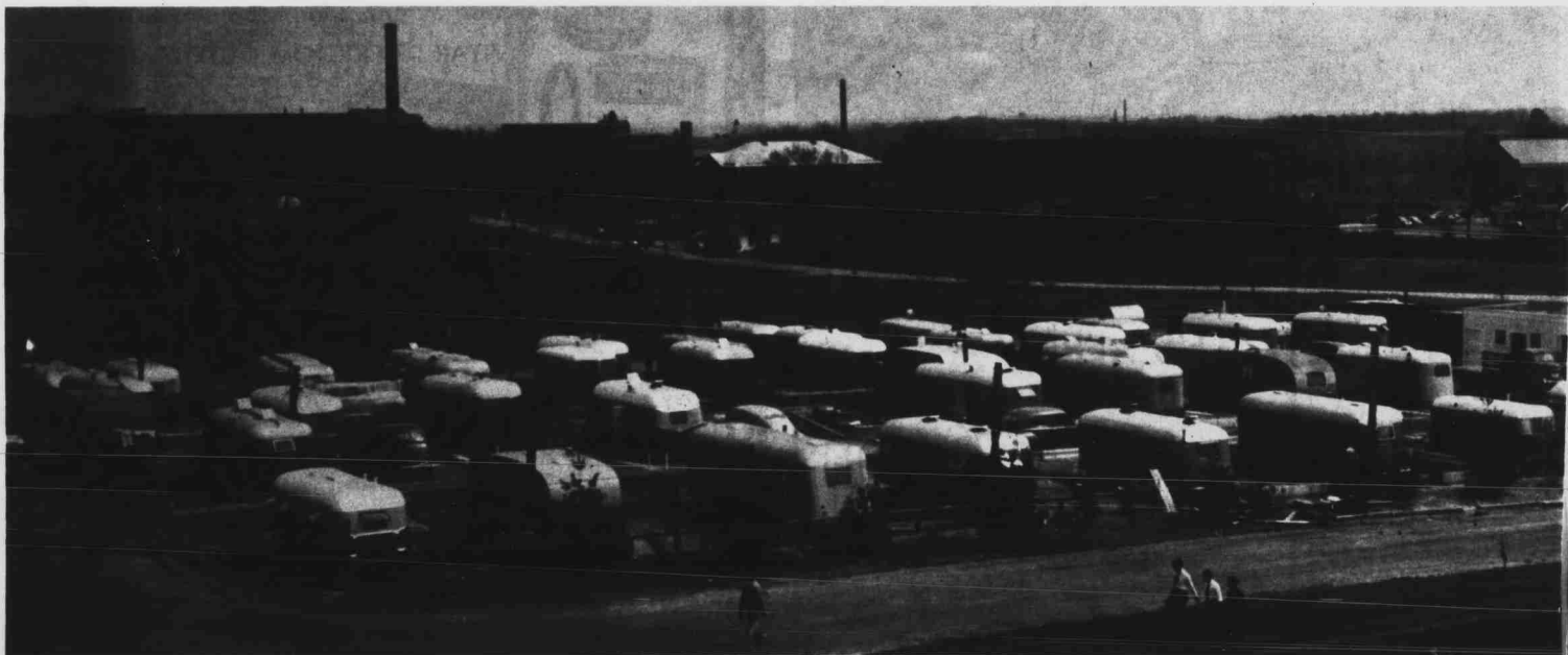
Trailwood was a trailer park for married students after World War II. It was located in the area of the brickyard. In the background, the steel framework of the Coli under construction.
