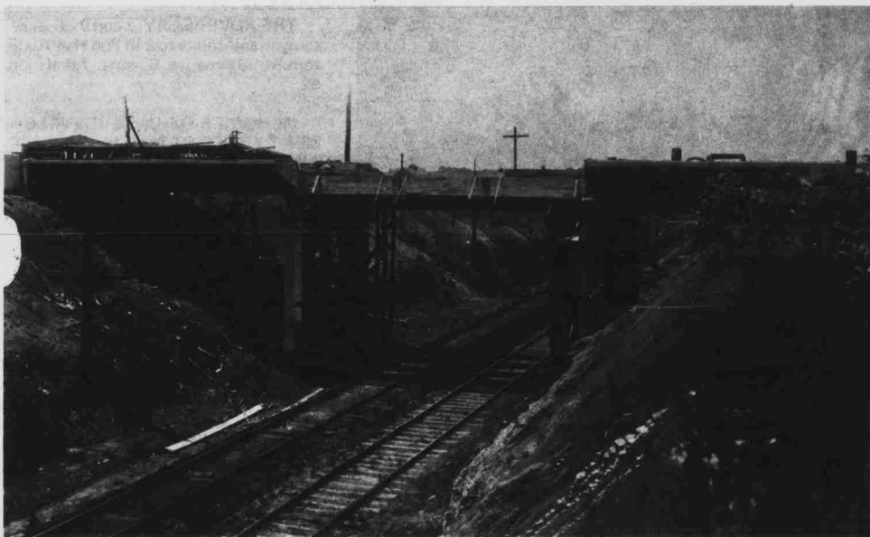
In July 1924 the Pullen Road Bridge was under construction. When the bridge was complete, it became a popular pastime of students to roll snowballs into steam locomotive smoke stacks.
