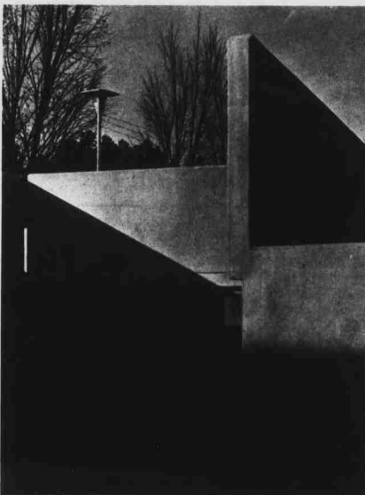
The Supply Store tunnel which was closed two years ago for the construction of the new Chemistry building will open shortly. See the story on page three. (photo by Hill)
