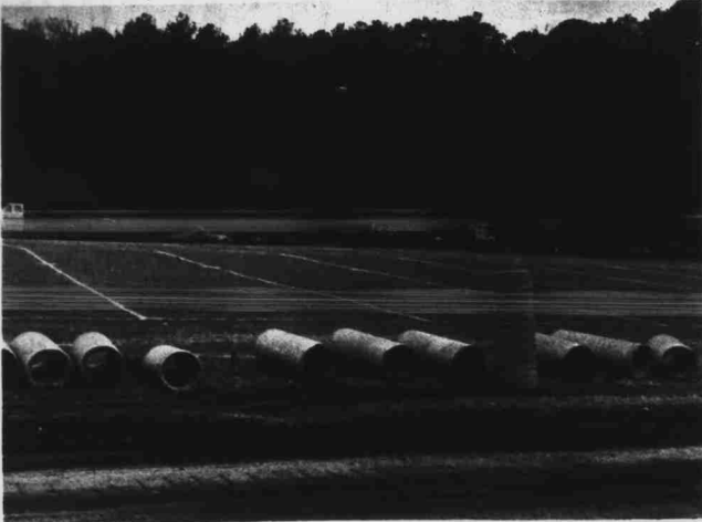
Construction has started on State's new nine-lane TarTan running track. Hopefully the new track, which will be one of the finest facilities in the area, will be ready in time for the fast approaching outdoor season. (photo by Barker)
