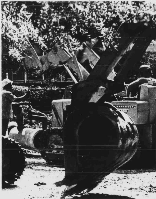
Construction began last week on the dorm landscaping project behind Bragaw Residence Hall. The project includes an amphitheatre and general landscaping of the area. (photo by Foulke)
