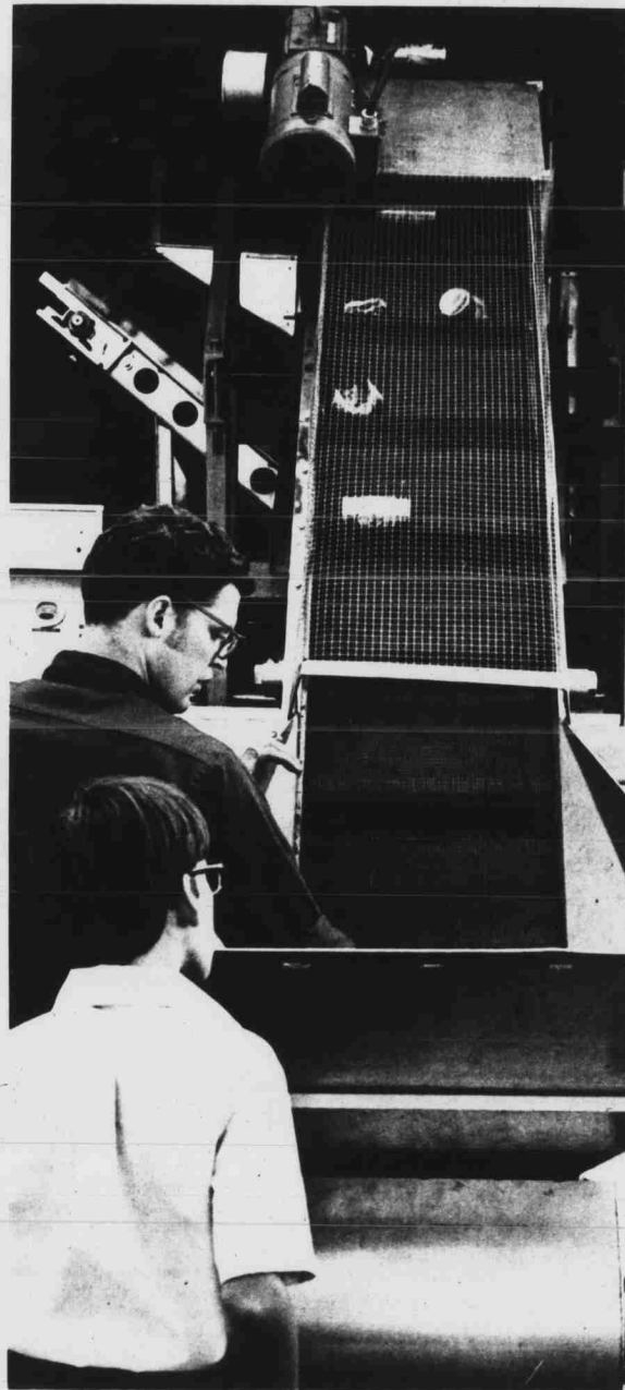
Recyclable aluminum cans, pie plates, butter tins are fed on a conveyer belt for feeding into the Reynold's Industry recycling machine.
