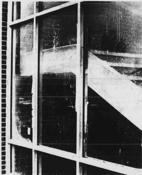
Vandalism hit the new Student Center this weekend even before its opening. Eight large plate glass windows were broken in the almost-completed building. (photo by Wright)
