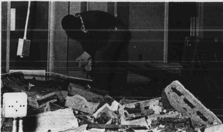
WALLS COME TUMBLING DOWN —Renovations have begun in the basement of the library. The wall in the old west reading room is scheduled to fall shortly. —photo by Cain
