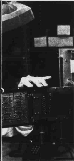
—photos by Cain electrical systems.
