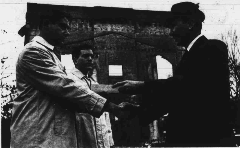
J. Perry Watson (right) receives a check for $60 from SPE President Frank Davis as former SPE President Buck Lee looks on. Demolition crews are in the process of razing the remaining two walls of Pullen Hall. (Photo by Sun Arreanu)
