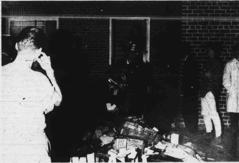
Firemen clean up damage in Holladay Hall following a fire believed to be caused by vandals. (Photo by Wooden)
