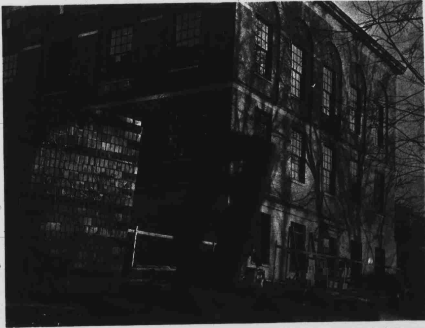
Technician Photographer Jerry Jackson caught this unusual picture of the Peele Hall renovation while touring the campus construction projects. Peele will soon be a Holladay Hall annex.
