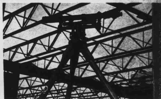
No, not the instrument of a forgetful CE class, but an interesting shot of the overhead beams in the multiple purpose room at the Faculty Recreation Center, only one of the many features of the Clubhouse. (Photo by Jackson)
