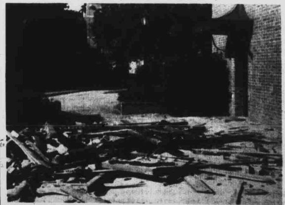
"That pile of trash in front was thrown off the roof of Watauga by the M & O as part of the remodeling job the dorm is undergoing. The door in the background is the Office of Information Services—whose employees are wearing steel safety helmets. The invisible hand sticking out from under the beams belongs to a student who blundered past the nonexistent guard rails and the imaginary warning signs.
