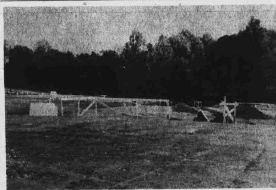
After years of breathless expectation on the part of students, work on Fraternity Row is finally getting under way. This is the site of one of the twelve houses now under construction.
