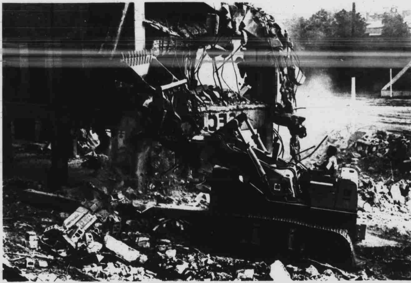
RIDDICK STADIUM FALLS—Demolition on the old stadium began last week. A bulldozer starts moving the twisted steel and concrete. The area will become a parking lot. (Photo by Overman)
