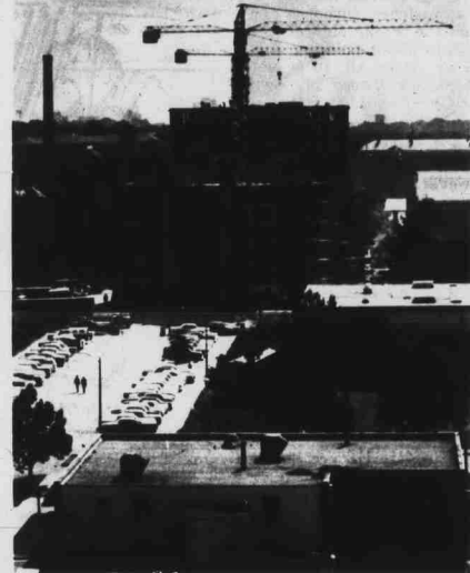
The rising trio of dorms on West Dunn Avenue will have all the comforts of home when completed. (Photo by Hankins)
