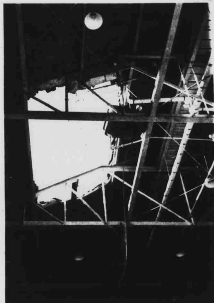
The stack's fall caused a 20 by 10 foot hole in the roof of the building and caused damage to several lights and a heater.
