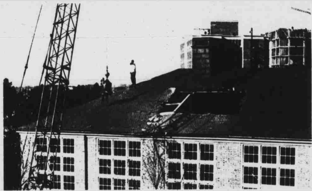
Monday afternoon a brick-lined, iron smokestack crashed through the roof of the Bureau of Mines Building when a crane's cable broke. There were no injuries in the accident. (Photos by Hankins).
