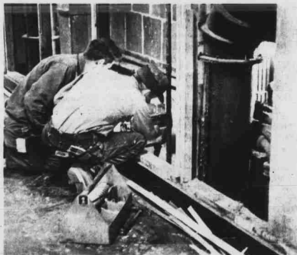
Labs in Withers Hall are being renovated to include modern hoods, electricity, and running water. (Photo by Moldov)
