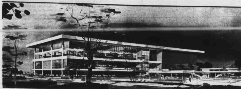
Construction on State's new $3.25 million Student Center should begin next Spring. The building will more than double the floor space of the present Union and be completed in 1970. (Photo by Hill)
