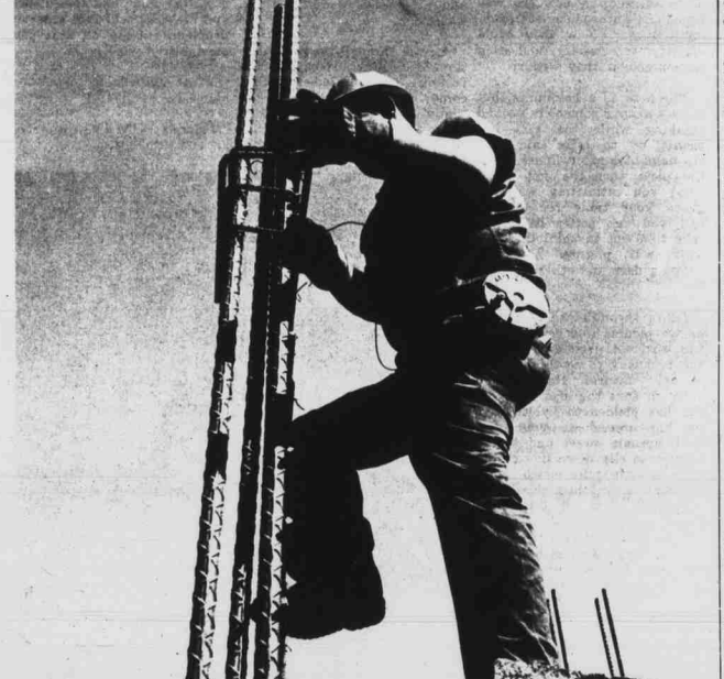
Construction, construction, construction. Work never seems to stop, whether it's a new chemistry building, new home for food science, or dorms for the coeds. The new structures for the campus reflect the changing personality—more room is needed for more students with wider and wider interests to investigate.
