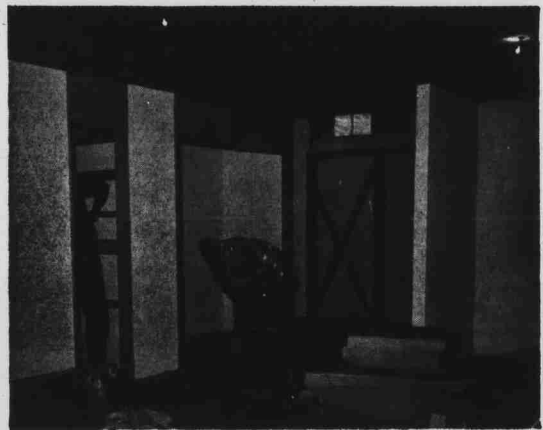
Progress continues on the new The Technician offices in the basement of the YMCA building. The space formerly allotted to the Student Supply Store will be converted to house The Agromeck , radio station WKNC, and the newspaper. It is anticipated that the move will be made during the summer months. (Photo by Kugler)
