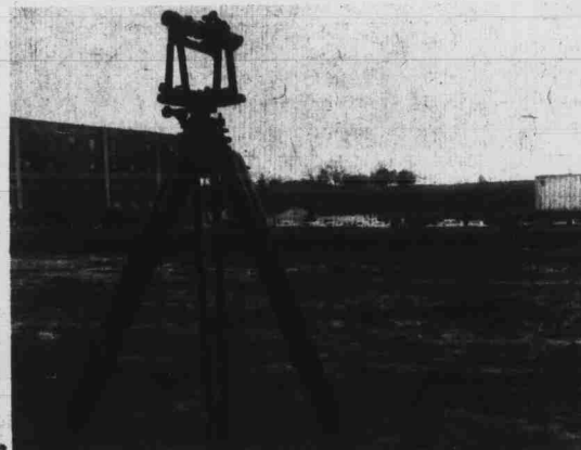
Work on the new cafeteria is beginning with excavation of the site between Tucker and Bragaw dormitories. The cafeteria will incorporate a new method of serving food, the Shuffle system. (Photo by Kugler)
