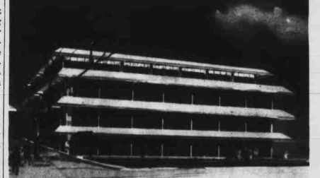
Construction will begin next year on the 1.5 million dollar addition to Kilgore Hall, housing the School of Forestry.
