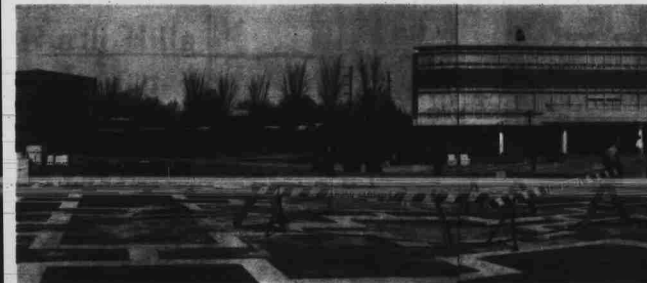
The sea of bricks has nearly been completed. Soon to come are shrubbery, floodlights, information boards, and benches. The Union-Harrelson landscaping project was a major undertaking; J. McCree Smith admits that it's more than his men can handle. Will it be left unfinished? (Photo by Hankins)
