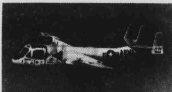
**MOHAWK**, a new observation plane on which production began in 1958—Grumman's first Army airplane—is designed to operate from small unimproved fields and will be used for purposes of tactical observation. Featuring a 59-knot stall speed and relatively the same short take-off and landing (STOL) capabilities as the Army's present light-weight single-engine airplanes, the Mohawk will be able to virtually "live" with the Army in the field.
