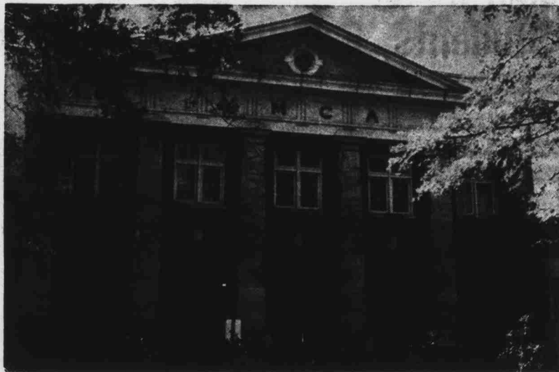
Home of Danforth Chapel
