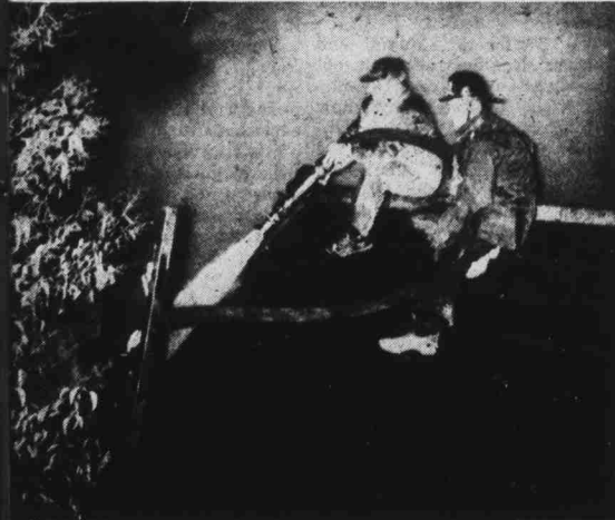
In order to keep the blaze from spreading to the residential section, firemen had to fight the fire from the roofs of garages.
