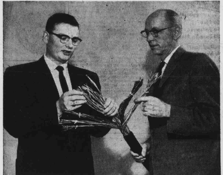
Stan Smith (left) discusses characteristics and color coding of polyethylene insulated cable with A. A. Little, Nebraska Area Transmission Engineer.
