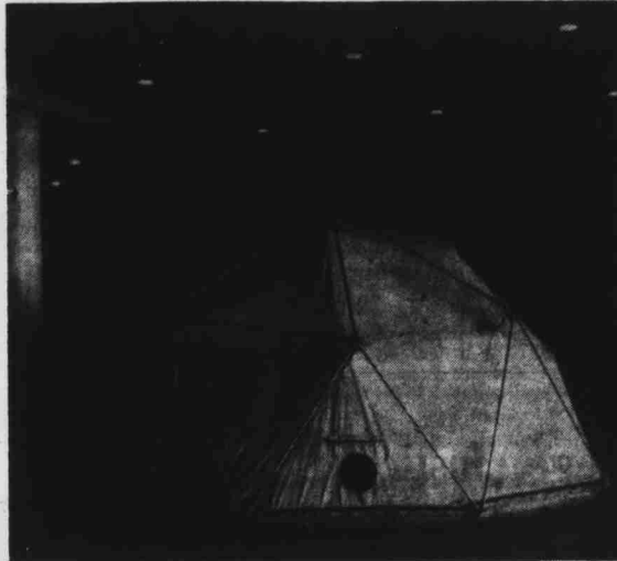
Shown above is a Geodesic Dome (It looks like a Volkswagen garage to us.) which is on display in the lobby of the College Union. The frame of the dome is made of magnesium and the membrane is made of coated nylon. (Photo by Kjosnes)
