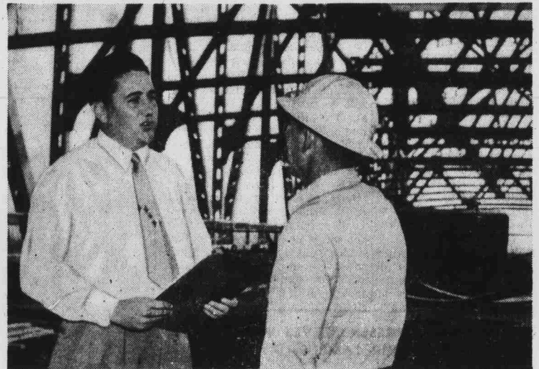
Bill Rhode (left) at the site of New Orleans' new Claiborne Street Industrial Canal Bridge.
