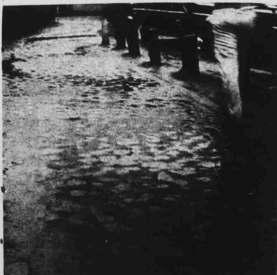
This is a sidewalk? Looks more like a mudhole. Shown above is the walkway leading to the Alexander-Turlington area.
