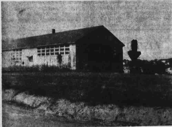
Above is pictured one of the broken down relics of the past on the State College campus. The building is now standing (barely) on the part of the campus along Western Blvd. The arrow to the right of the building points to the new 800-man dormitory now under construction. The building overlooks the campus from the south. We think it is an eyesore to the campus and should be torn down.—Photo by Barnhardt.
