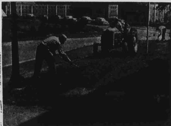
State College's new lighting system was well on the road to completion when the above picture was taken. Shown above are two men of the crew who are involved in burying the conduit for the circuit which is being laid without breaking up the sidewalks or streets. Two types of lamp standards are being used, tall posts for streets and the conventional posts for courts. The project is slated for completion the last of this month. (Staff photo by Wall)
