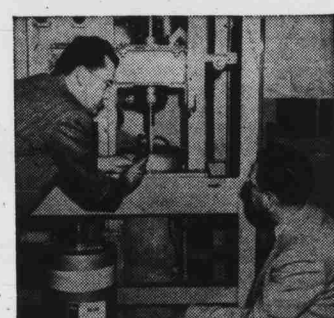
W. A. Hawkins (left), B.S.M.E., Carnegie Tech., demonstrates extrusion of "Teflon" tetrafluoroethylene resin for a customer.
