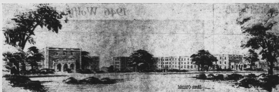
These two buildings pictured above are the new dormitories already under construction just on the other side of Alexander and Turlington. They are being built through a loan secured by the
