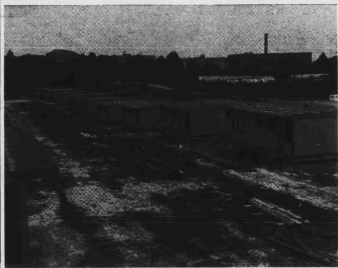
FUTURE HOME FOR VETS —Shown above are part of the 352 emergency apartments now under construction on the campus. Contract was awarded to the J. A. Jones Construction Company of Charlotte. This is an attempt to remedy in part crowded conditions on the campus.
