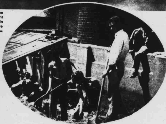
Looking Ahead — This construction gang is part of a botany class at Washington College, Chestertown, Md., making an enlargement to the greenhouse as part of their class project. Such work provides good training for the military job that is ahead of the boys.
