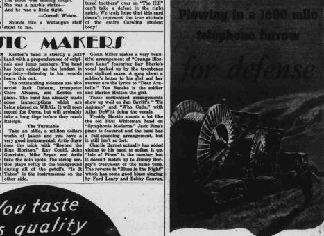
Several newly developed "plow trains," working from opposite ends of the line, are burying the cable for maximum protection. They dig deep furrows, lay two cables in them and cover them with earth—all in ome continuous operation. Their meeting will mark completion of the first all cable line across the continuous. ms will be operated in the cables ransmission in each.
