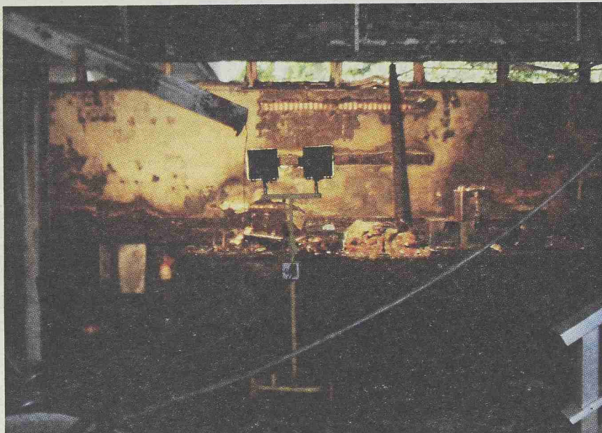
Tuesday's fire caused major damage to the Coffee Shop inside the Atrium food court. Photo courtesy Randy Lait
