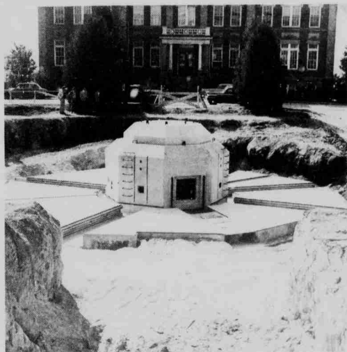
(Below) The nuclear reactor under construction. In the background is the Animal Industry Building, on the present site of Mann Hall.
