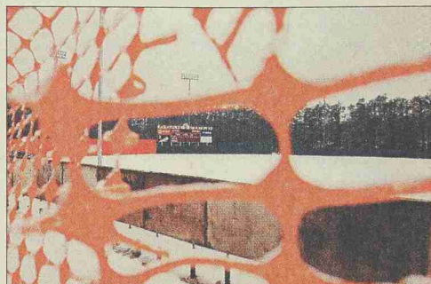
Construction on Doak Field has caused the displacement of DW parking spaces. The general contractors hope to finish the work before the end of spring. Staff photo by Matthew Huffman
