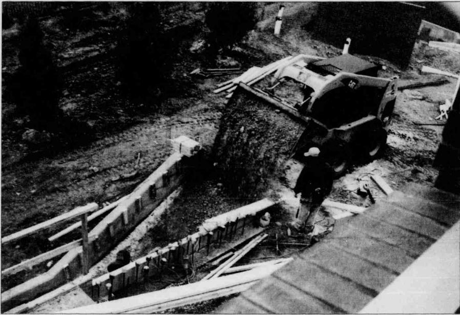
Ground broke on the new TKE fraternity house last summer and the new TKE house will open with a ceremony the first week of July.
