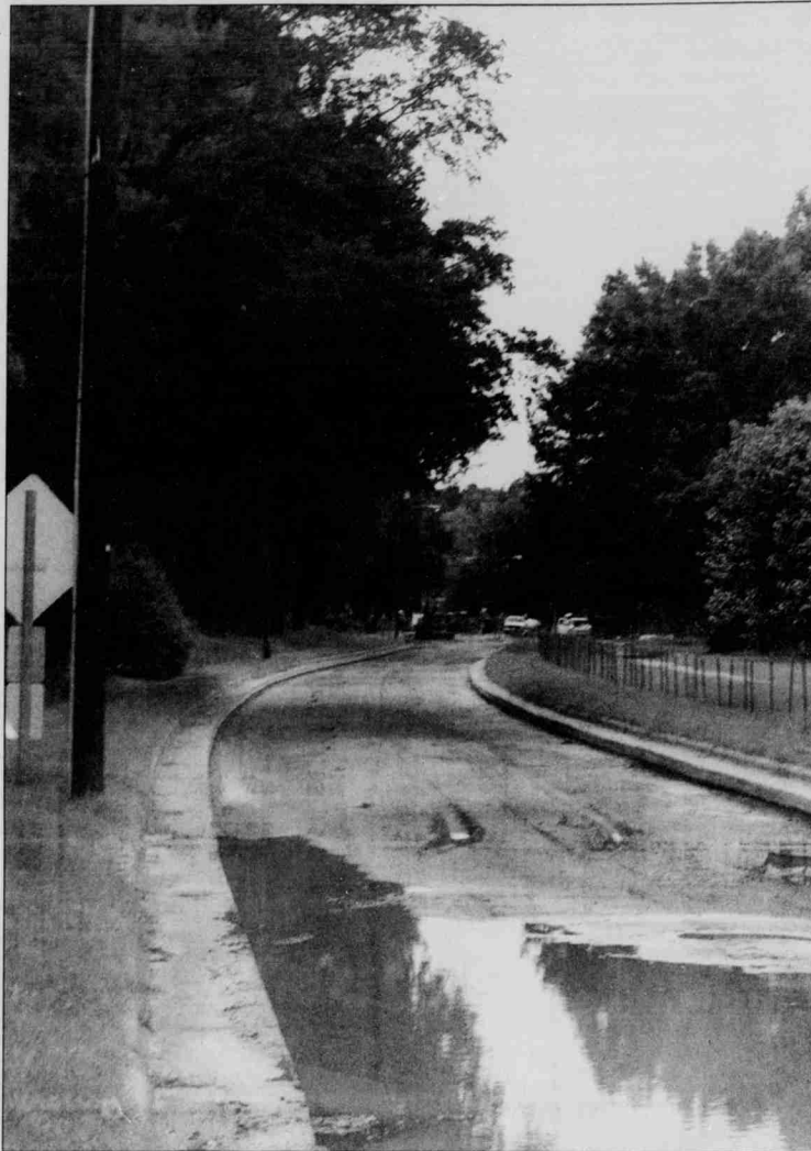
The continued construction on Sullivan Drive will likely be completed by the time students return to campus for the fall semester.
